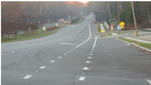
New acceleration and deceleration lane for the entrance of Admiral's Ridge on Route 2
